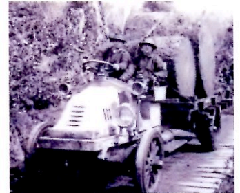
Moving two veneer blocks in the early twentieth century (Pacific County Historical Society)
