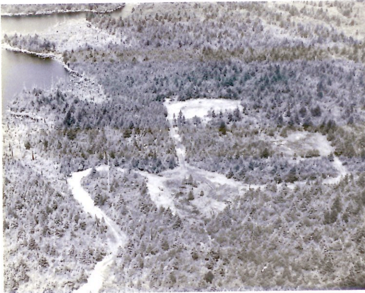
Construction begins on the new campus in the spring of 1963.
