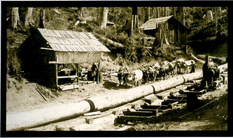
The combination of a bull team and a narrow gauge rail line made for excellent production when the timber was located some distance from a river or slough. Note the log carts behind the homemade locomotive, and how the logs are “sniped” or beveled on the end to prevent hang-ups when skidded by the bull team, circa 1895. Coos Historical and Maritime Museum, Jack Slattery Collection 992-8-0380
